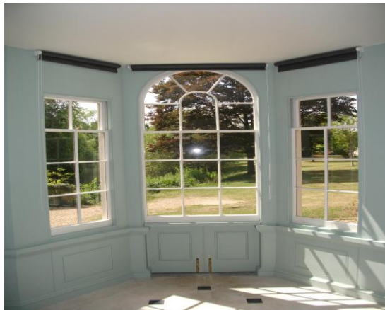
Restoration of gazebo in Langtons Gardens by Historic Buildings and Landscapes Officer, with the support of Friends of Langtons Gardens
